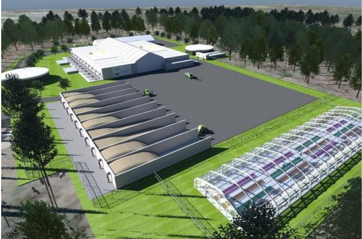
Figure C.7: Turning Earth Central Connecticut's Three-Phase Integrated High Solids Dry Fermentation In-Vessel Composting facility model, Southington, CT (from Turning Earth, 2014, used with permission).
